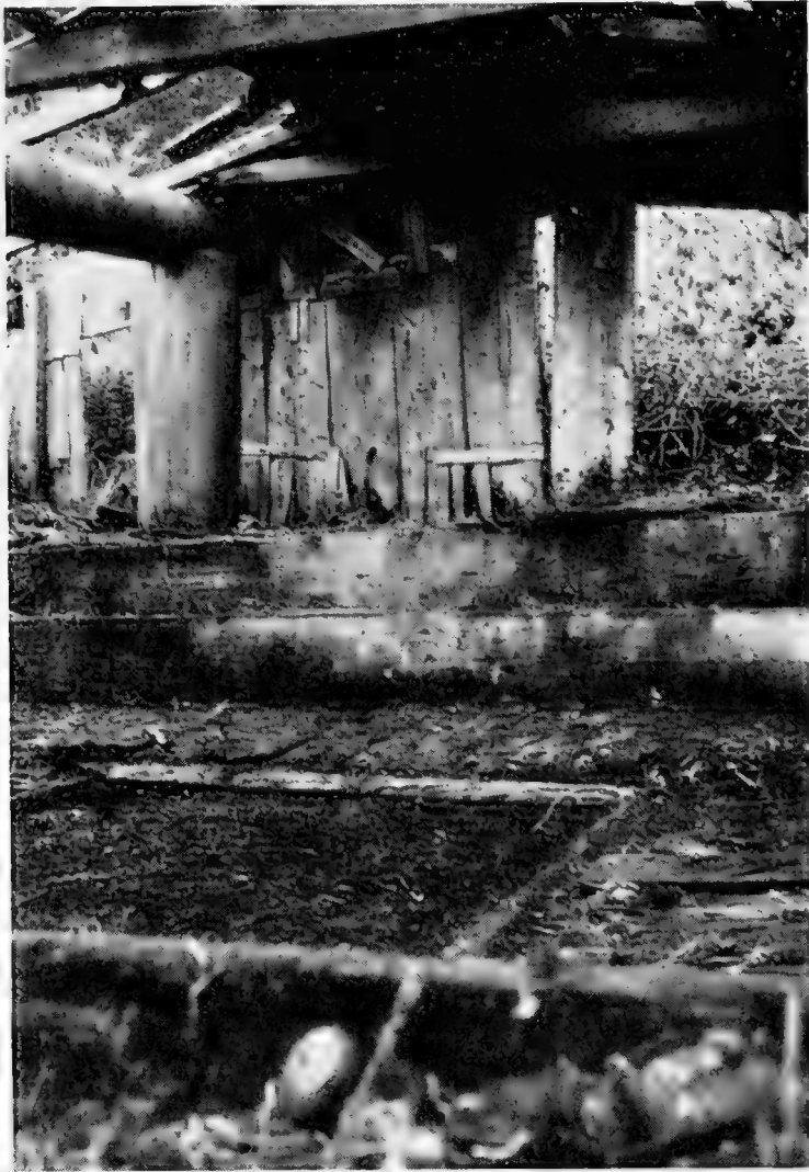
FIG. 180.—Interior of Eagle House. Two benches or floor levels rise on each side of the centrally excavated pit. The hearth is at the center of the pit, and the remainder of the floor including the two benches is covered with split cedar slabs. See figs. 177-179.
